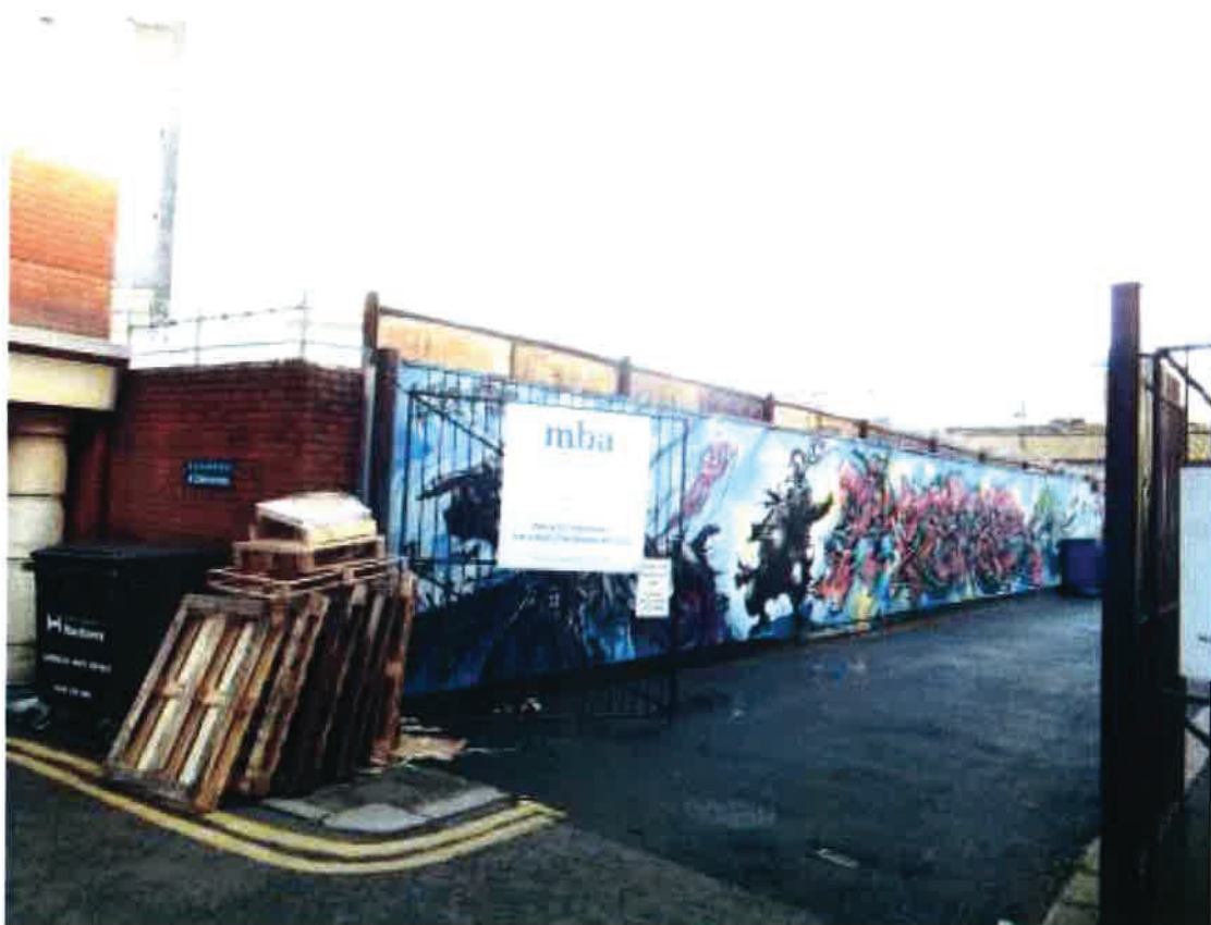
Figure 2: Rear view of site from Hewlett Street (site behind hoarding)
